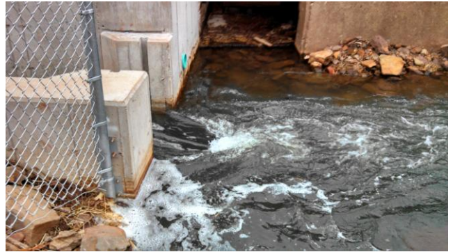
Above: the entrance of the StanChem fishway, showing good attraction water conditions for migrant fish. The entrance to the eel pass is seen in the background (the green pipe in the wall). The entrance net has not yet been installed in the eel pass but will be installed soon.
